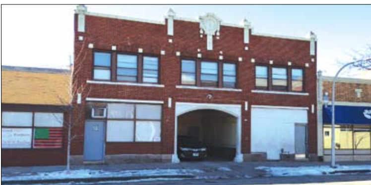
Once renovated – without the carport – New Life Interim Shelter will house 40 individuals who are homeless or in immediate crisis. Neighbors, partners, churches, and others have donated supplies and are involved in fundraising to rejuvenate this much-needed emergency shelter.
